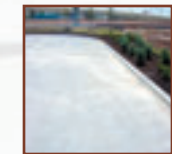
Light colored pavement
